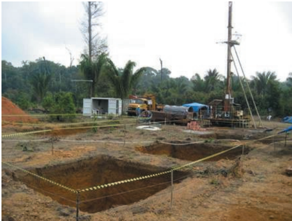
Brazil Potash – Drill hole in progress
