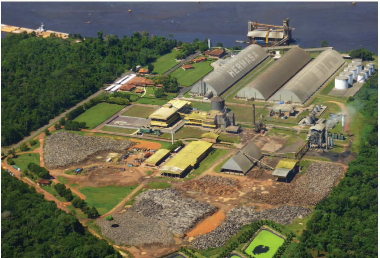
Brazil Potash – Logistics facilities near Manaus
